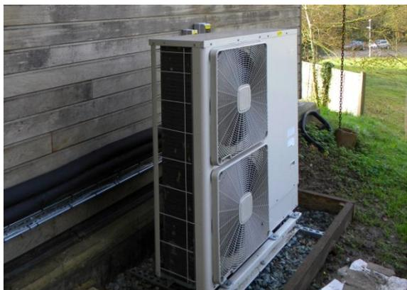
**Figure 2** The newly installed air source heat pump
